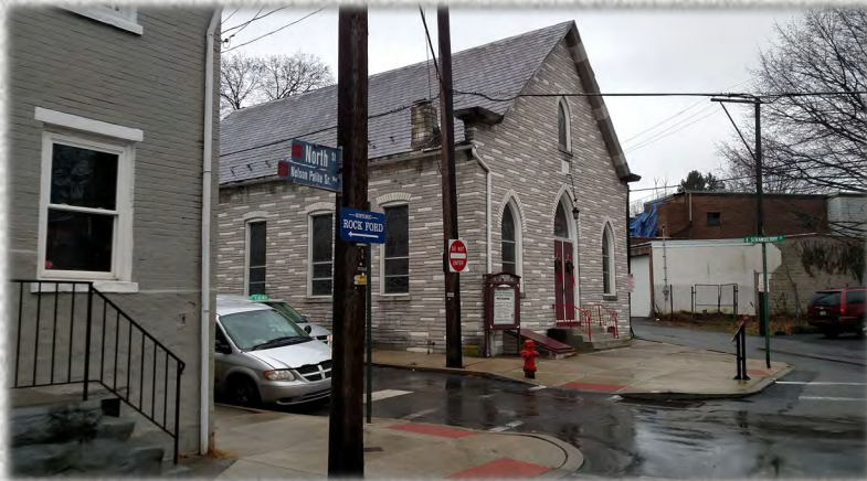
Bethel African Methodist Episcopal Church, Strawberry & North Streets View from North Street near Polite Family Home
