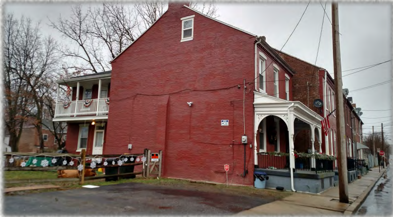
540 North Street-Southwest elevation
